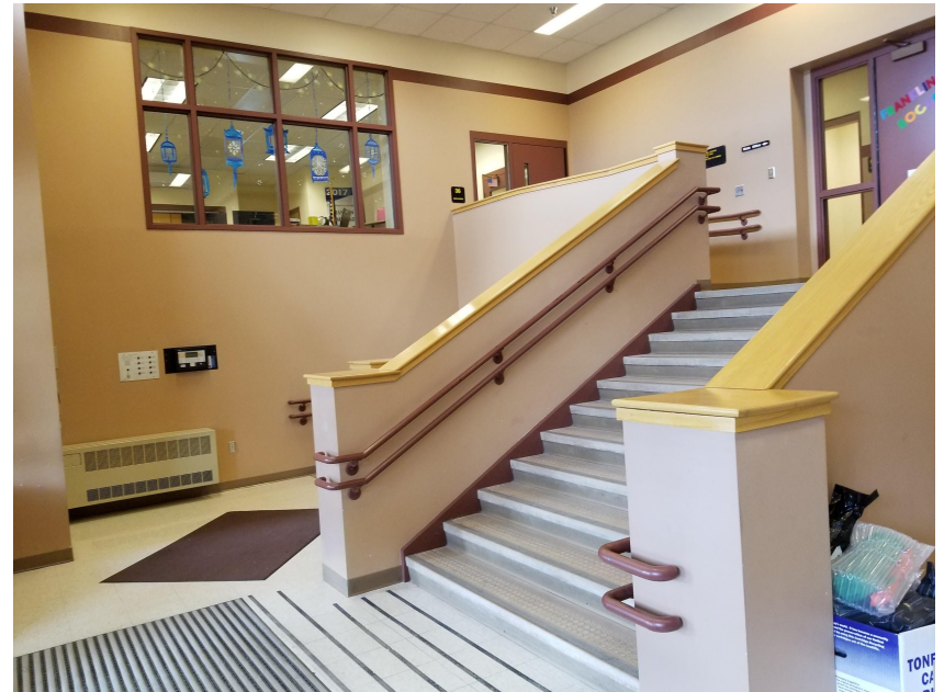
Main Entrance Stairs
