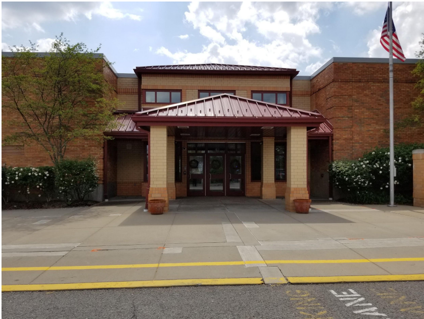
Existing Main Entrance
